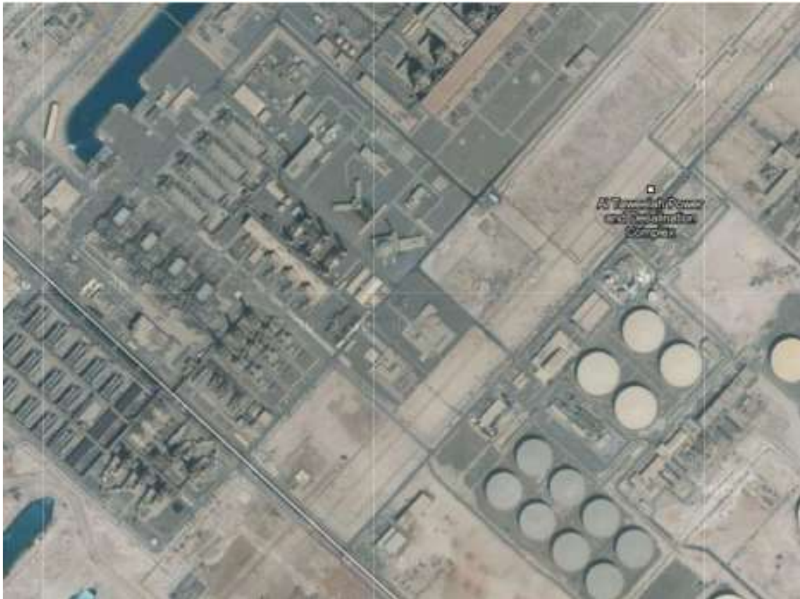
Figure 22: Key Target Examples: Gulf Desalination Plant
